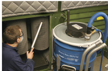
A clogged filtering system for a buffing booth is quickly cleaned and put back into service using the Heavy Duty HEPA Vac.
